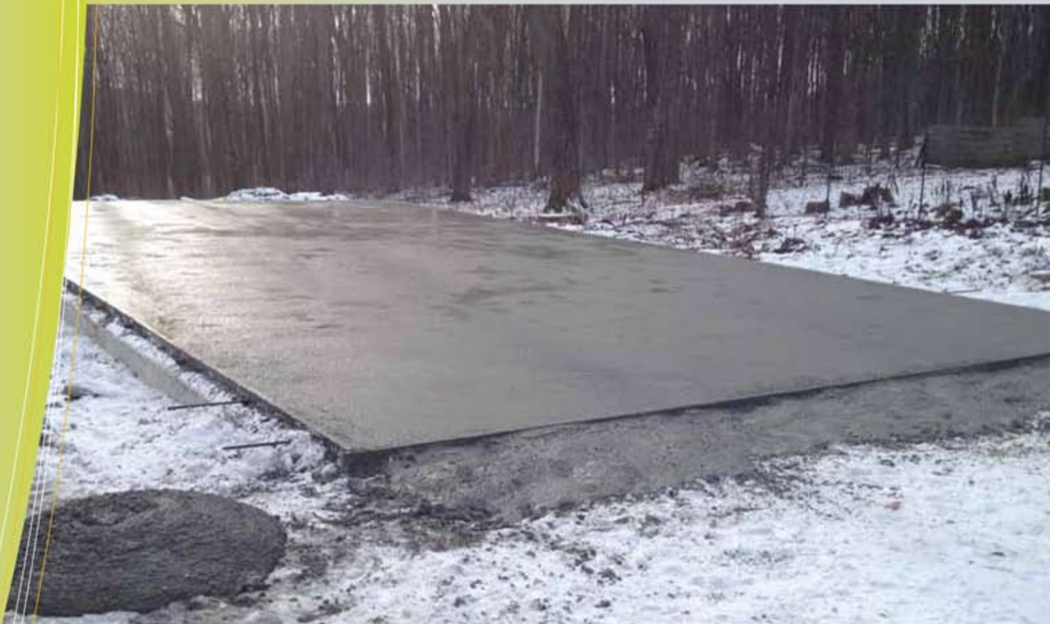
“MK5 Foundations Salvage Damaged Foundations”
