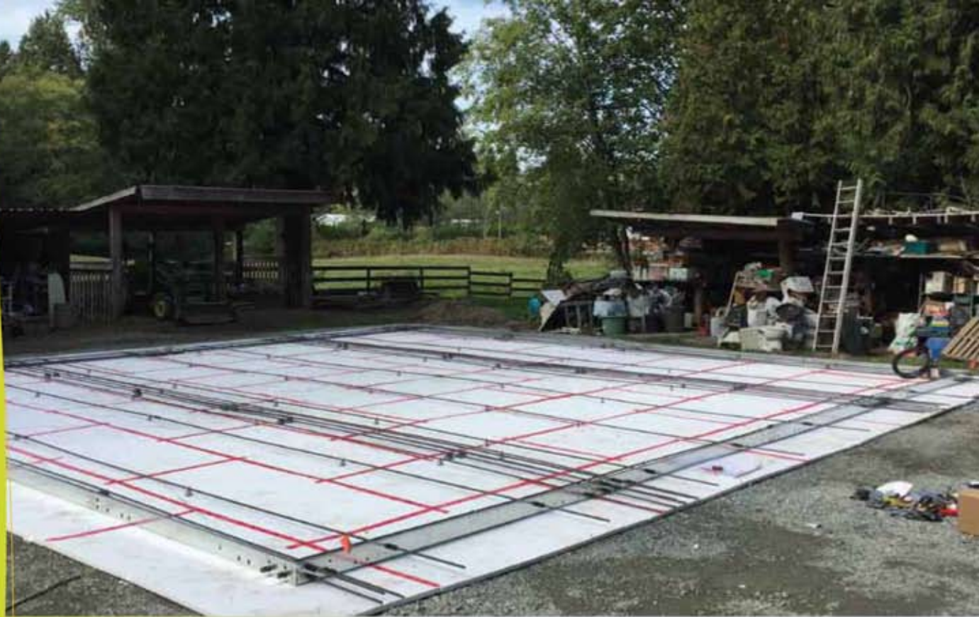
“MK5 Foundations Float Multi-Span Frames”
